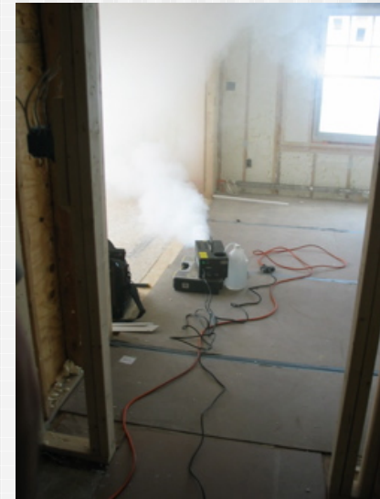
Test all installations before drywall
